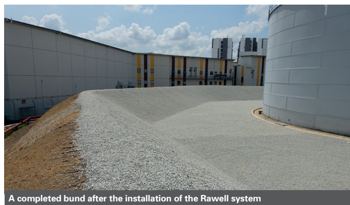
Rawdrain is laid over the Rawmat before the stone backfill is placed
