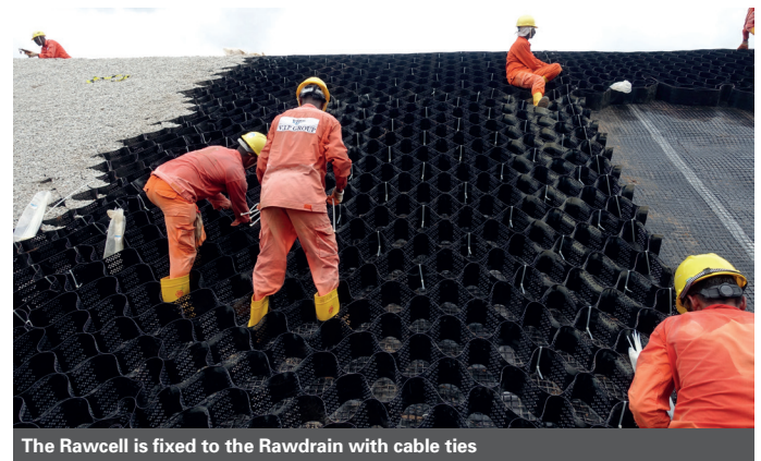
The Rawcell is fixed to the Rawdrain with cable ties
