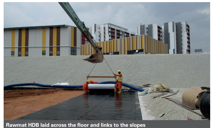
Rawmat HDB laid across the floor and links to the slopes
